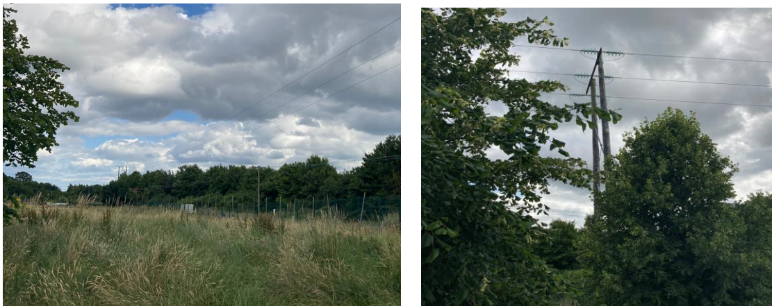
Figure 5. Existing 38kV line traversing the site
